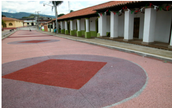
Figure 3-5 Example of Ecocreto Installation in Soyalo, Chipas, Mexico
